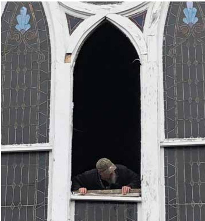
A workman removes damaged stained glass window.
