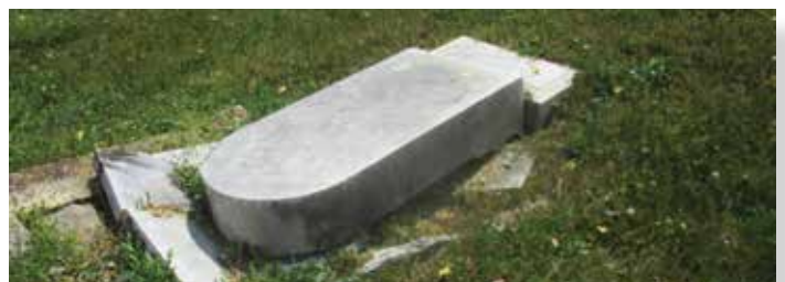
One of several stones off its base and on the ground.
