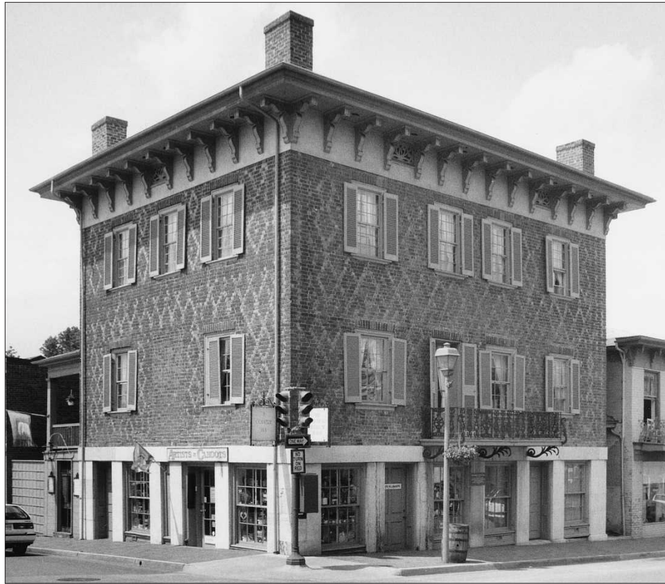
The Alexander-Withrow House at the northwest corner of Washington and Main Streets, after restoration. Note the distinctive diamond-shaped brick pattern. Photo courtesy of the Virginia Department of Historic Resources.
