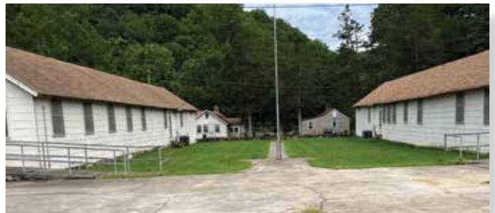
Housing from the CCC camp is being restored and renovated.
