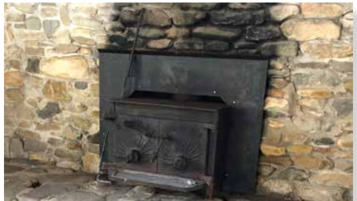
A well preserved CCC era fireplace.
