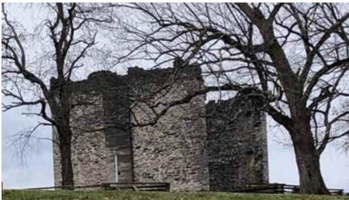
The c. 1793 Liberty Hall Academy House ruins. Photo Credit: HLF
