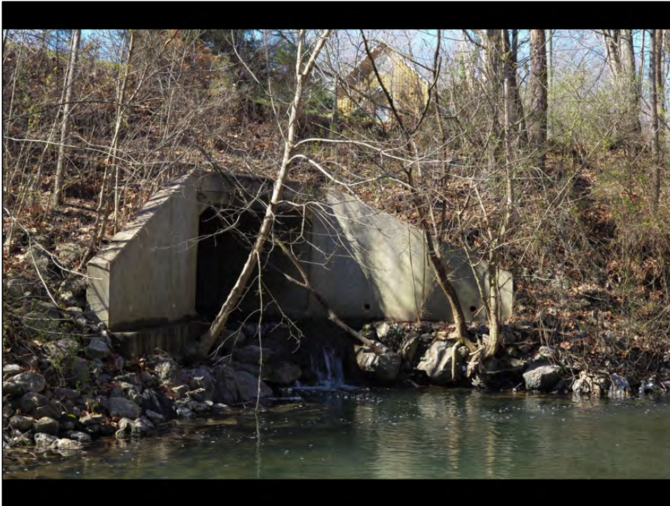
directly below Beechenbrook Chapel (visible above culvert)
