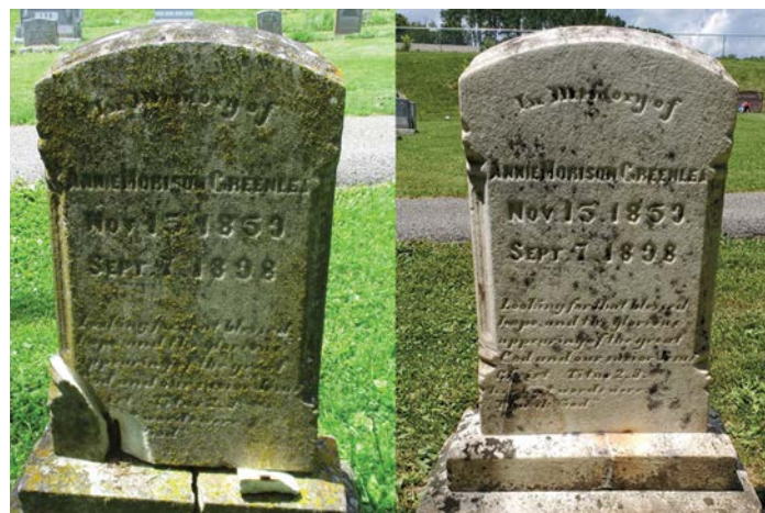
Gravestone in Evergreen Cemetery of Annie Morison Greenlee. Left: Broken at metal pin and broken base. Right: Repaired.
