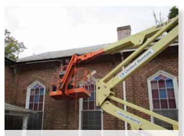
Welsh Construction workers remove the gutters and replace fascia board in preparation for the installation of new gutters.
