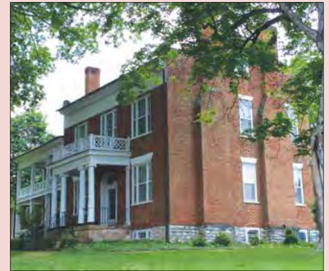
Reid-White-Philbin House today from West Nelson Street (above) and from Barclay Lane (top left); staircase photo courtesy Library of Congress.
