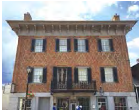
North Main Street façade.
