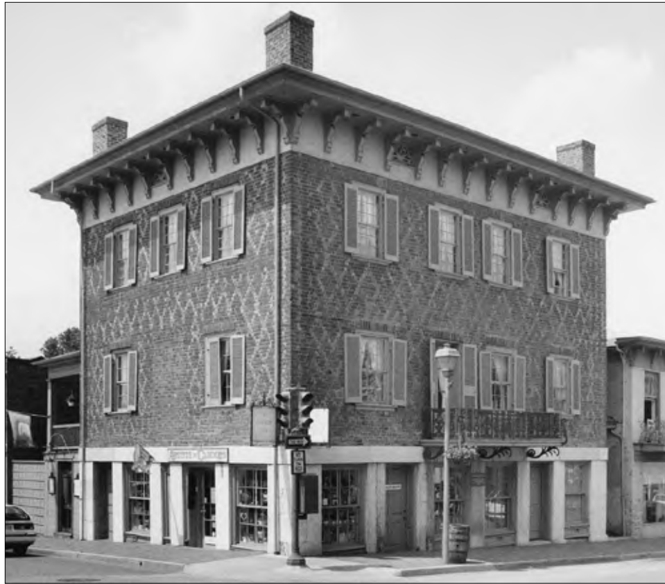
The Alexander-Withrow House at the northwest corner of Washington and Main Streets, after restoration. Note the distinctive diamond-shaped brick pattern. Photo courtesy of the Virginia Department of Historic Resources.
