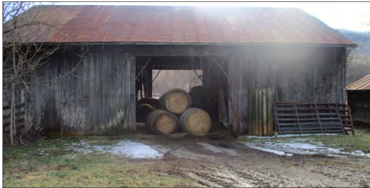
Double-bay drive-through barn
