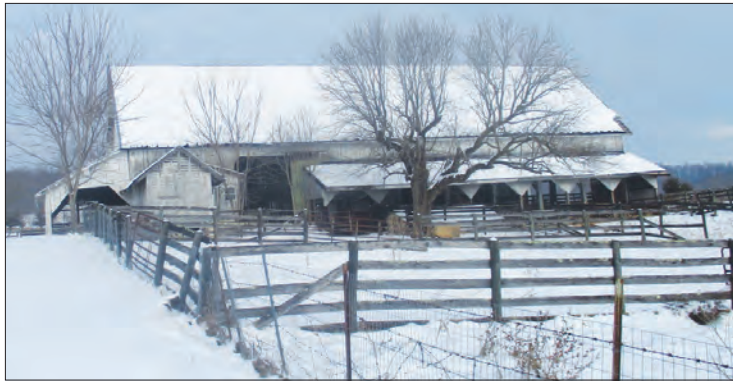
Double-bay drive-through barn
