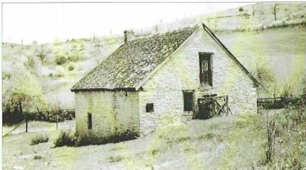
The Stillhouse at Willson Farm, also called Tuckaway, has now been completely demolished.
