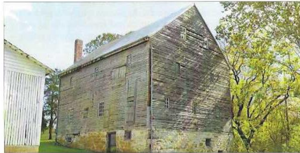
Also known as Steele's Mill for William Steele, who owned the property in 1819, this structure is typical of stone and timber construction used in industrial buildings in rural Rockbridge County. It is also included in the National Register.
