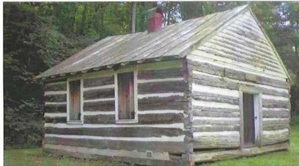
The Hamilton School, listed on the National Register, is one of the last old log field schools built before the Civil War in Virginia. Built by the community on land conveyed by Robert Hamilton, the log structure also served as a church.
