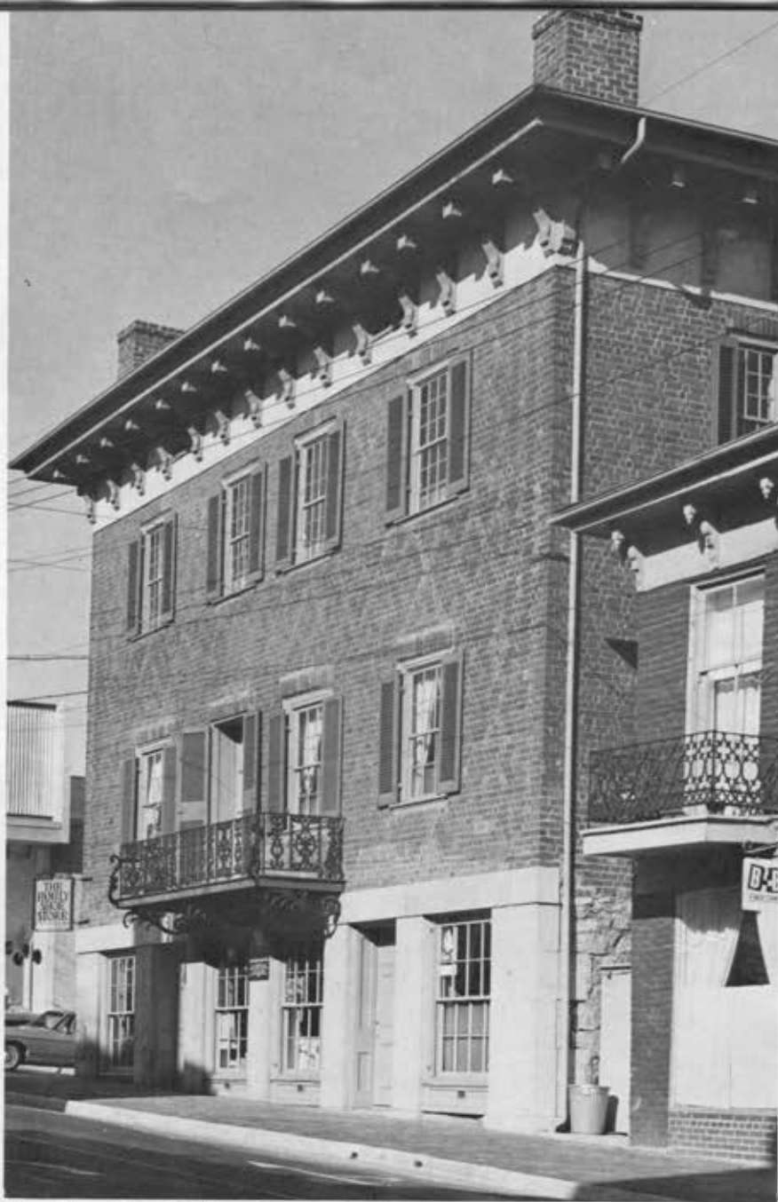
The Alexander-Withrow House, built 1789. Note diamond brick patterns.
